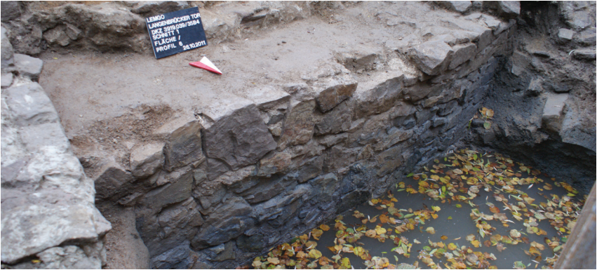
Figure 3: Northern abutment of the bridge.
